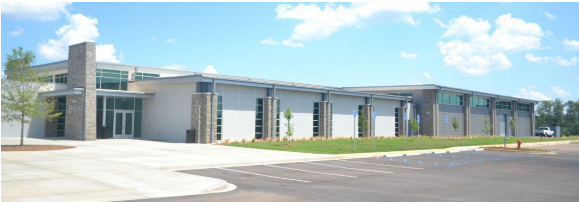
The new Tri-County Technical College facility in the Oconee Industry and Technology Park.
