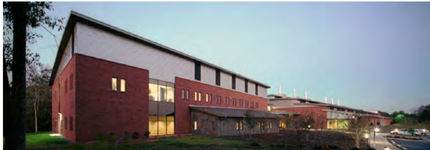
Clemson University's Advanced Materials Center in Anderson County. Photo credit: Clemson University.
