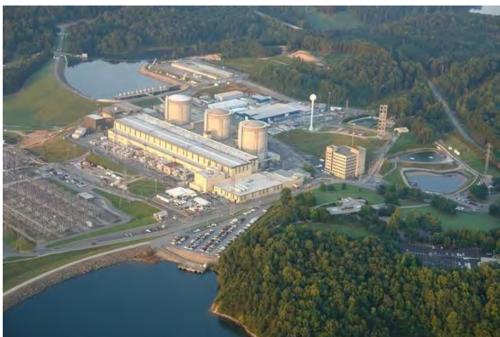
An aerial view of Oconee Nuclear Station in Oconee County. Photo credit: The State Media Company
